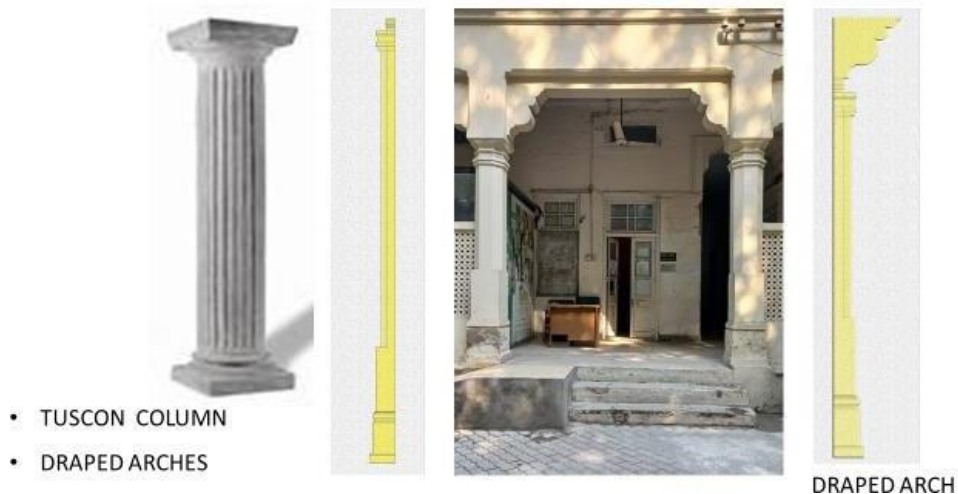
Figure 14: DETAILS OF COLUMNS IN GANGA RAM BUILDING Source : Author
